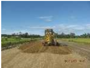
Spreading aggregate base class B. (Km 80+000 - Section 4) 19 Apr 2011
