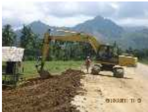
Trimming embankment slope (Km 83+100 - Section 4) 20 Apr 2011
