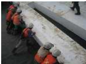
Installing geofoam at Lambeso south approach (Km 82+600 – Section 4) 31 May 2011
