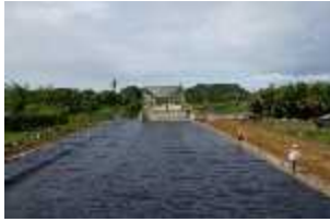
Placing geomembrane for Lambeso north approach (Km 82+600 - Section 4) 01 Jun 2011
