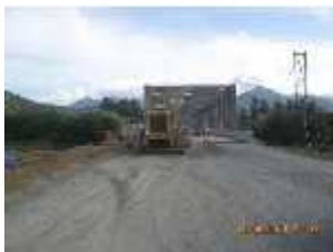
Spreading aggregate base class A at Lambeso Bridge (Km 82+675 – Section 4) 20 Jun 2011
