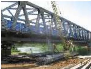
Installing pedestrian rail for Lambeso north span (Km 82+600 - Section 4) 02 May 2011
